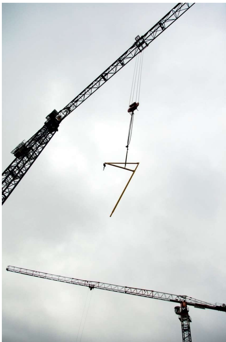
Example of handling of rotary arm with crane
