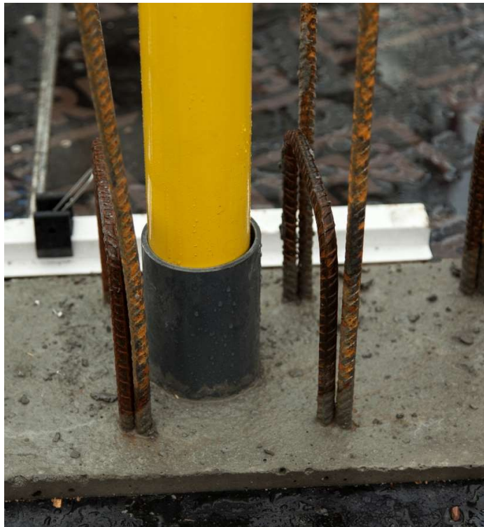
Rotary arm after embedding in socket
