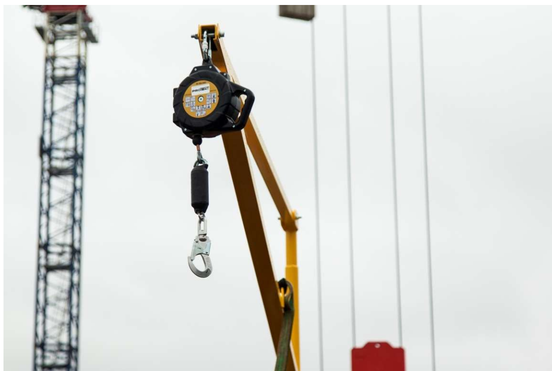
Connection of retractable type fall arrester to rotary arm
